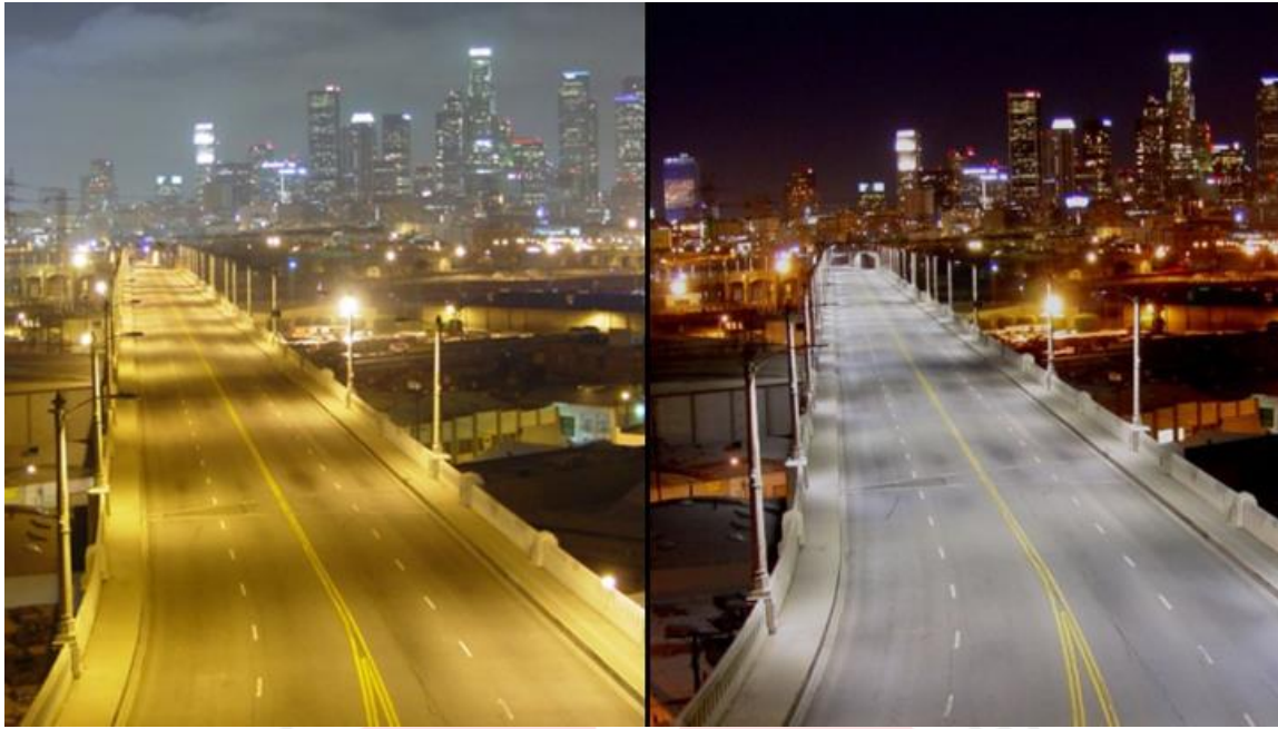
Figure 4. Road illumination under yellow and white light
