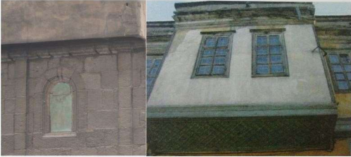
Fig. 5. Ground floor made of cut stone and first floor covered with plaster
