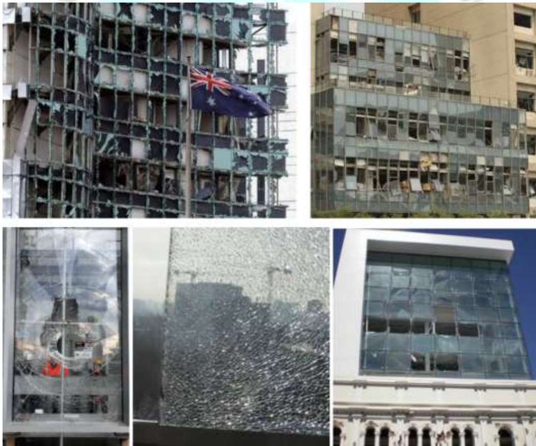
Figure 2. Different Failure Types of the CWs ([13], [14])
